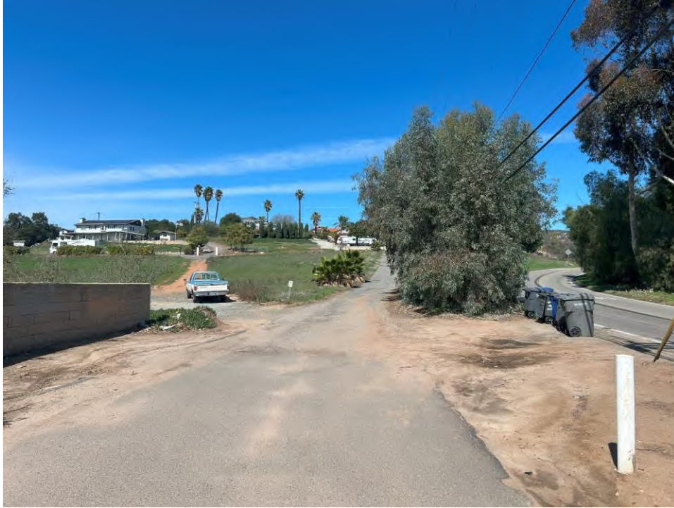
Photograph 2. View of laydown yard from intersection of North Broadway and North Avenue. View north.
