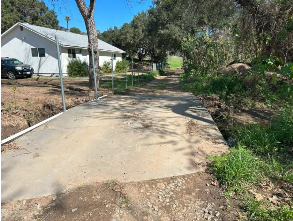
Photograph 6. View of Kellrae Lane bridge over Reidy Creek. View east.
